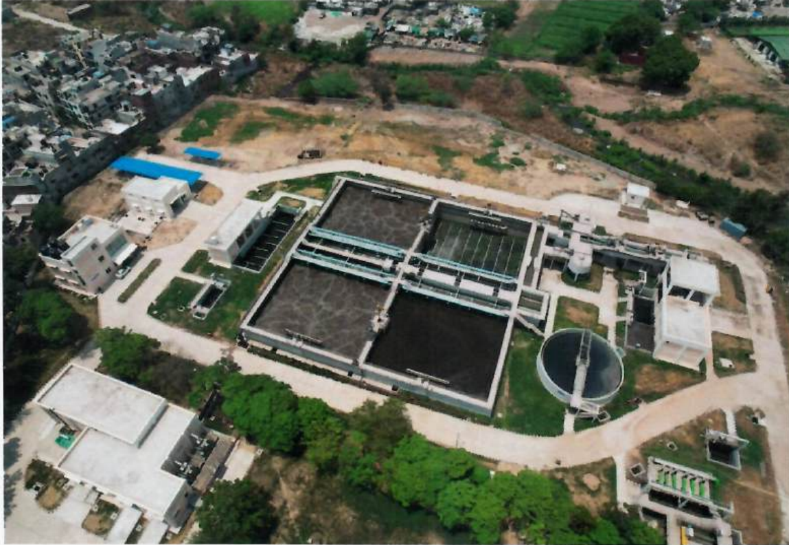
STP RAIPUR KALAN - I
